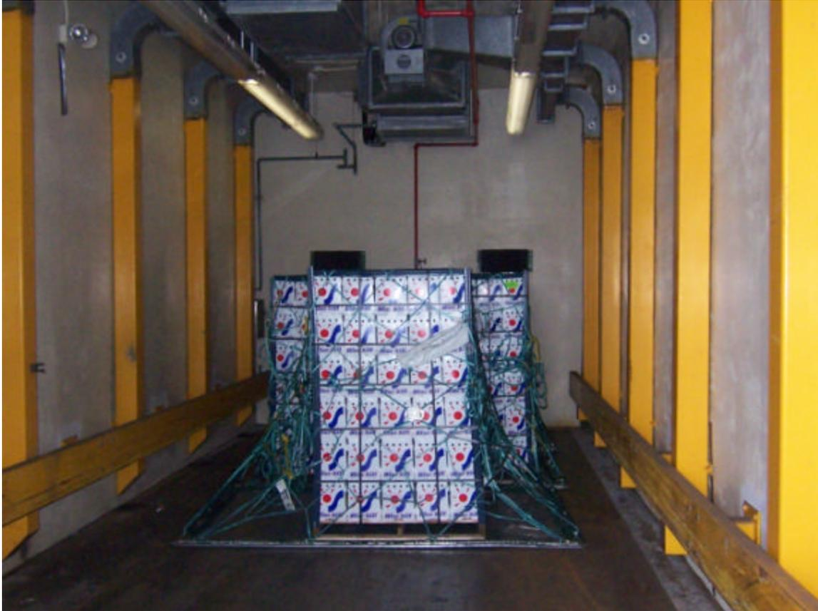
**Fumigation chamber at Atlanta Hartsfield International Airport. Asparagus just arrived from South America must be fumigated before shipment to distributors. Chamber is approximately 4,300 cu ft and has internal circulation fans.**
